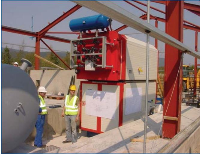
*A 400 kW biomass boiler: Biomass boilers work best for community-wide schemes, where they can operate with a largely constant load. Where they are used within a building, they benefit from being procured by a fully integrated project team, with client and specialist supplier on board early, that fully considers the post-occupancy operation and management issues not just theoretical technical performance.*
