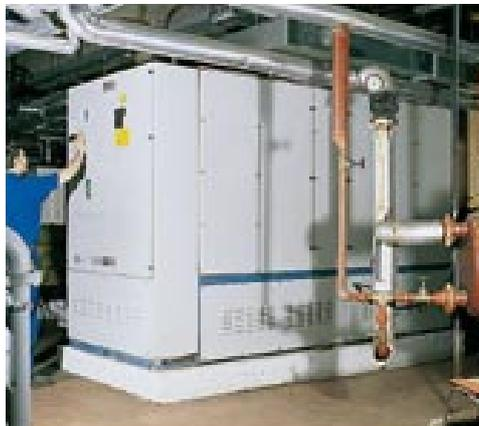
*CHP plant at Huddersfield operating as the lead boiler*
