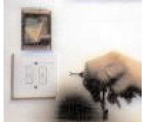
*'Fish tail' switches allow lights to be switched on and off by staff using a special key*
