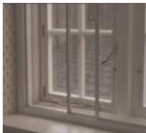
*A layer of glazing has been added to these opening casements - improving their performance while maintaining their external appearance. Sliding secondary glazing has been provided in the window reveals*
