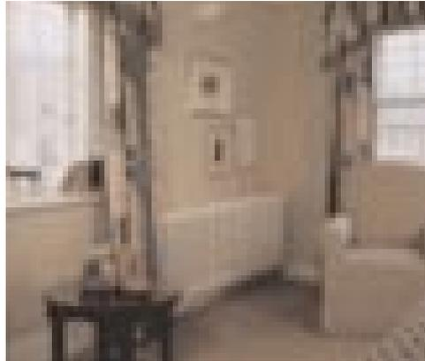
*Radiators are positioned to avoid being obscured by curtains at The Calls, Leeds. These walls are dry-lined with insulation-backed plasterboard*
