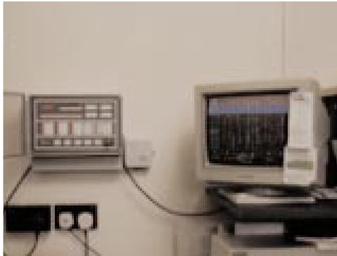
*The control panel for operating guest room heating from reception is positioned next to the room-booking display screen at The Calls, Leeds*
