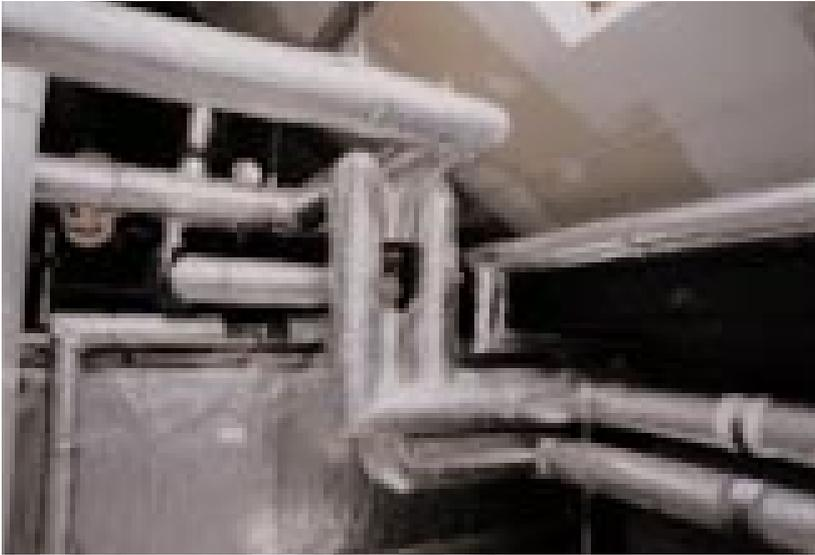
*Pipework and tank insulation. Note the labelling of tank and service pipes*
