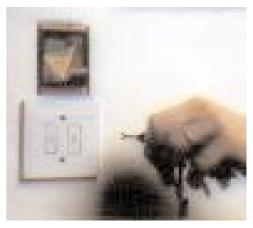
'Fish tail' switches allow lights to be switched on and off by staff using a special key
