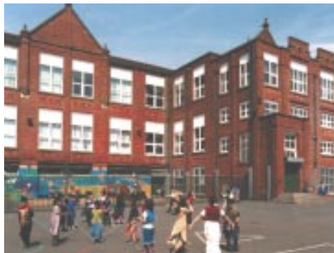
Figure 9 Sunning Hill Primary School, showing the new windows on the south façade
