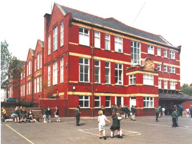
Figure 1 Church Road Primary School
