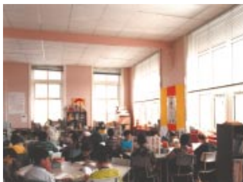
Figure 10 Suspended ceilings and new windows reduce heat losses at Sunning Hill Primary School
