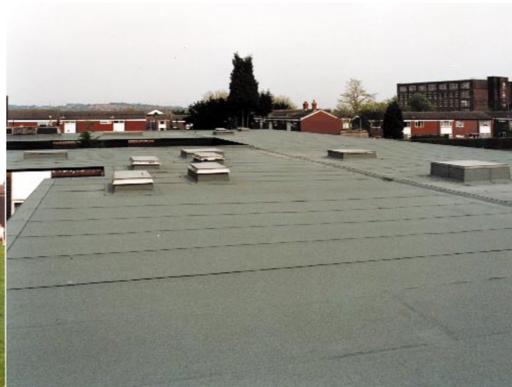
Figure 12 The new insulated roof at St Matthew's Primary School
